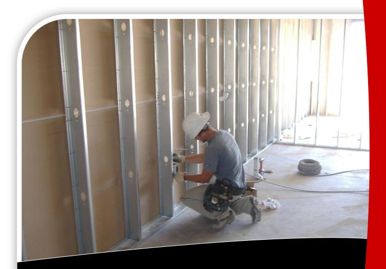
PRE-FAB ELECTRICAL WIRING ASSEMBLIES
