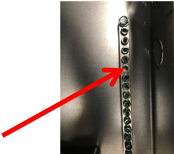
4. Replace the grounding bar and secure both screws in the mounting holes. Torque the screw in the extruded hole (provided with the panelboard, #1 shown below) to 25 in-lbs, and torque the self-threading screw in the drilled hole (#2 shown below) to 15 in-lbs in order to properly bond and secure the Ground Bar to the panelboard enclosure.
