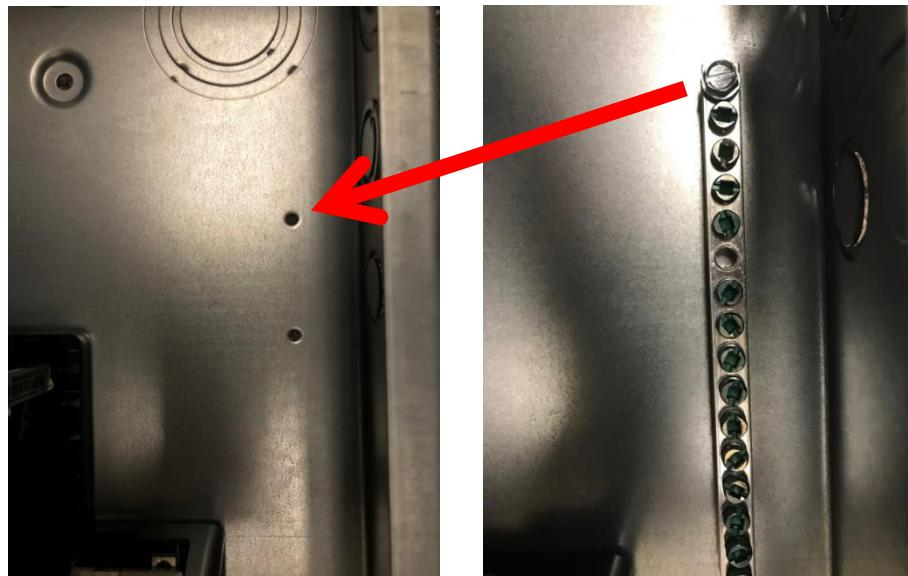
3. With the Top Screw threaded into the enclosure, use the Ground Bar as a template by positioning it to establish the desired drilling location of the mounting hole (as shown below). Mark the desired hole location and remove the bar. Using an 11/64" drill bit, drill the mounting hole. Ensure that spacing requirements are maintained according to NEC® Table 408.56 and remove all metal shavings and debris inside the panelboard (loadcenter) enclosure.
