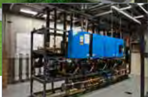
Parallel refrigeration rack (C)
